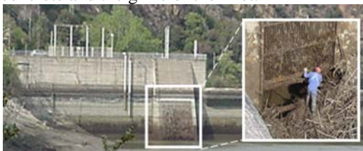
Fig. 2 Vegetal residuals obstructing the water inlet of Pasteral Dam in Girona.
